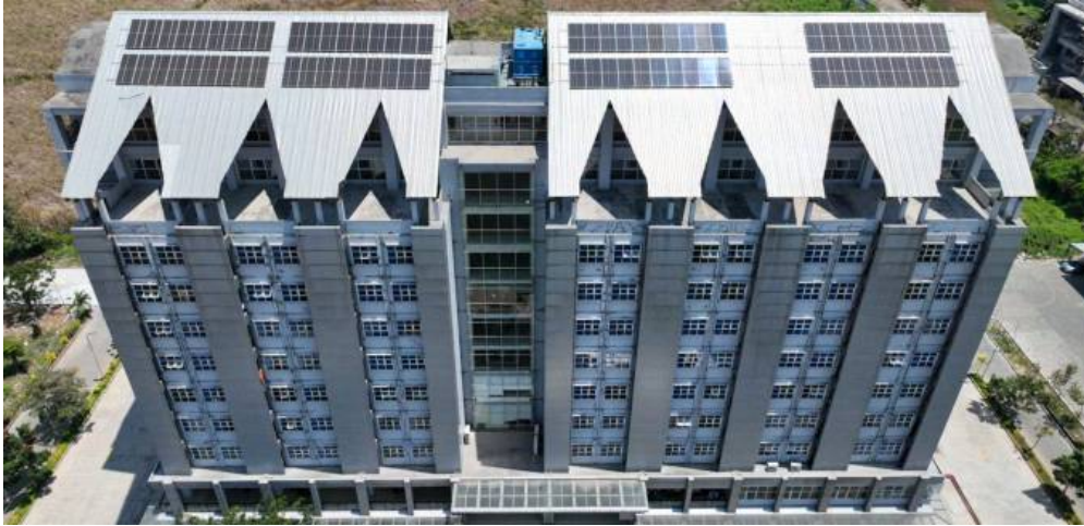
Figure 10. Solar Panel in Rooftop of Female Dormitory UNAIR Source: Directorate of Facilities and Infrastructure, 2024
