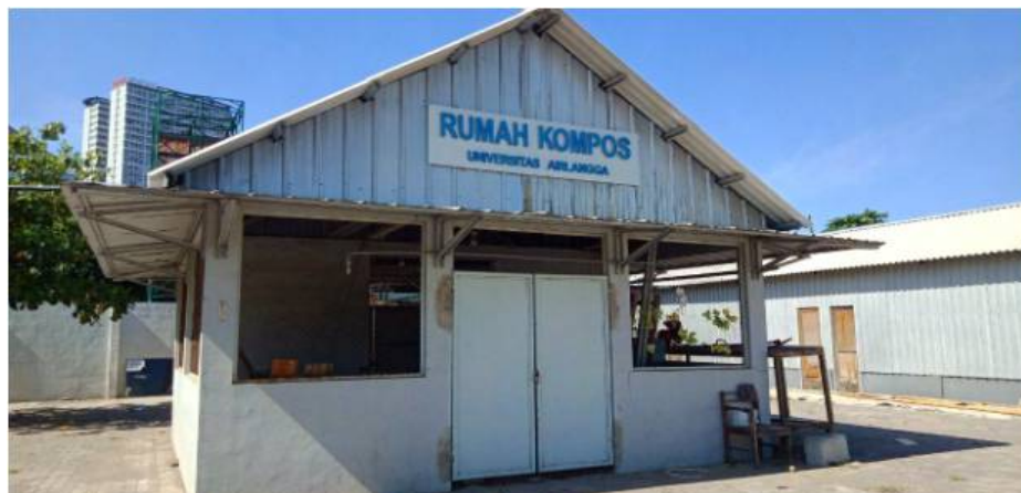
Figure 25. Compost House UNAIR
